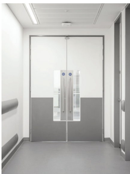
Antimicrobial copper door furniture installed at Francis Crick Institute. Courtesy of Allgood.
